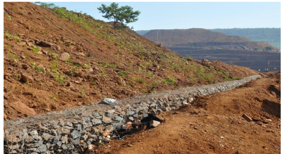
Retaining wall at dump-3
