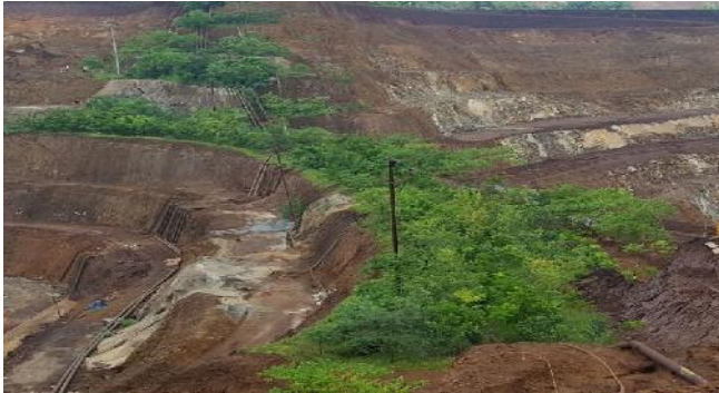
Vertiver Plantation and Grass Turffing at Dump slope
