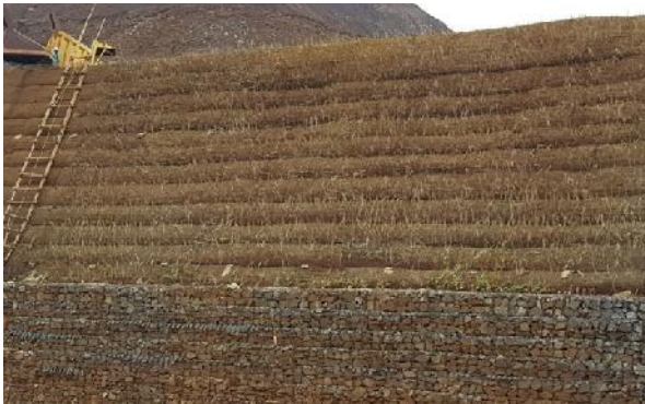
Vertiver Plantation and Grass Turffing at Dump slope
