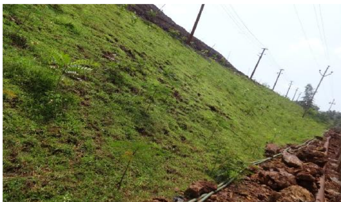
PHOTO-10: SHOWING GRASS TURFING OVER DUMP SLOPE
