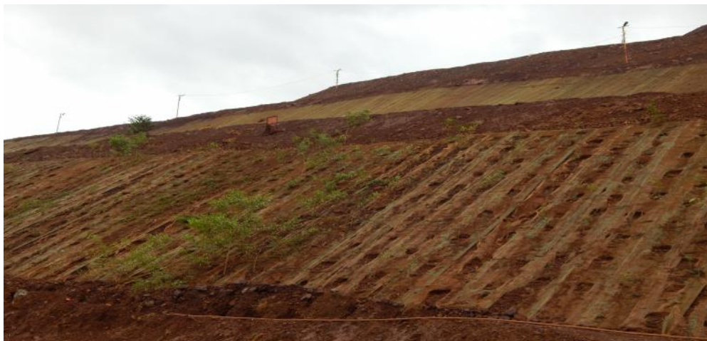
PHOTO-10: SHOWING GRASS TURFING OVER DUMP SLOPE
