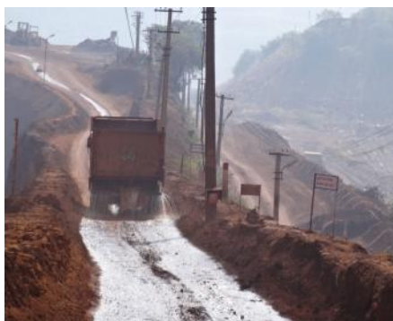
PHOTO-6 : SHOWING MOBILE SPRINKLERS INSIDE MINES
