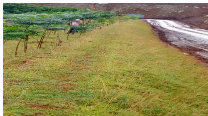
PHOTO-10: SHOWING GRASS TURFING OVER DUMP SLOPE
