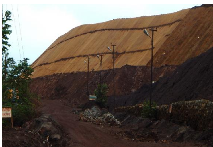
PHOTO-9: SHOWING COIR MATTING OVER DUMP SLOPE
