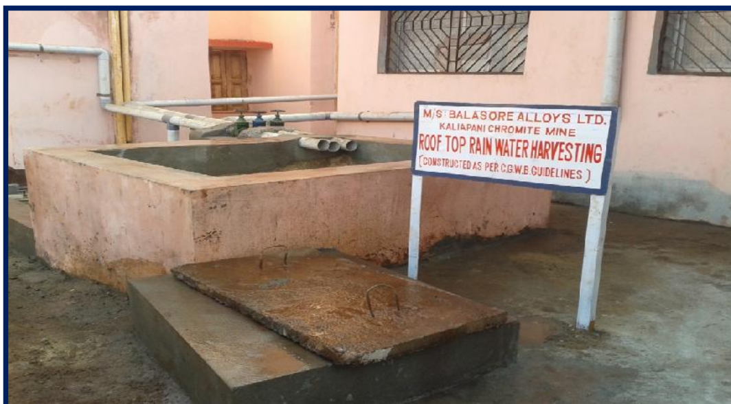
PHOTO- 7: SHOWING ROOFTOP RAIN WATER HARVESTING STRUCTURE
