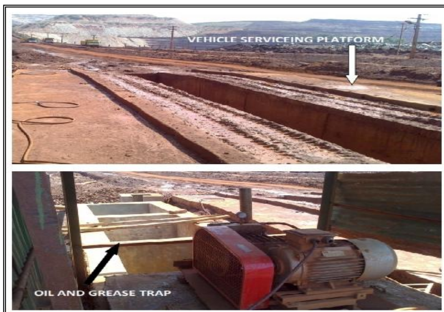
PHOTO-18: SHOWING VEHICLE SERVICING CENTER WITH OIL & GREASE TRAP
