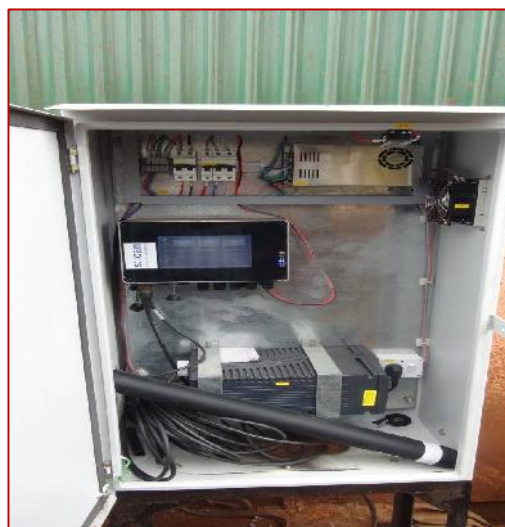
Photo-02: On-Line Monitoring System installed at In-let & Out-Let of ETP
