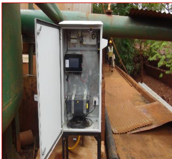
Photo-02: On-Line Monitoring System installed at In-let & Out-Let of ETP
